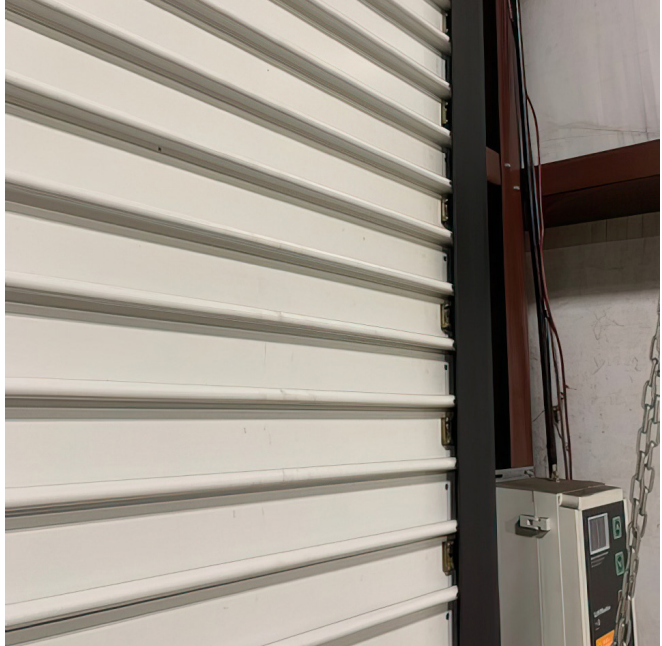
Figure B6: Rolling Door, Non-Insulated – Interior View Shows Slat Cavities
