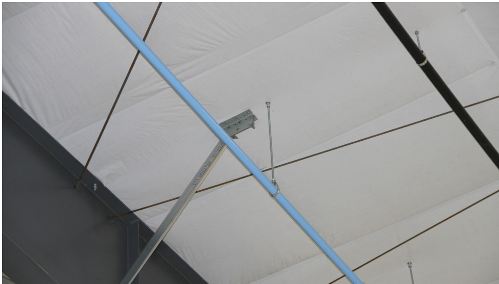
Figure 17: Flange Brace and Pipe Hanger CAB Options
