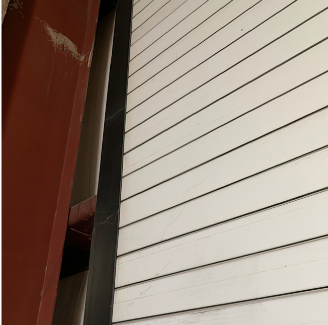
Figure B5: Rolling Door, Insulated – Interior View Shows Smooth Surface
