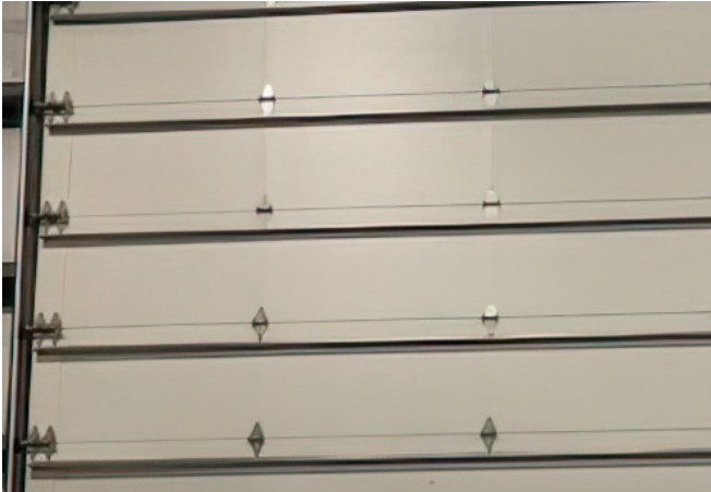
Figure B3: Sectional Door, Insulated – Interior View Shows Flush Surface
