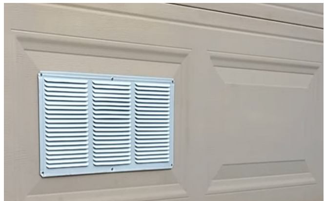
Figure B17: Sectional Door – Vent (a.k.a. Louver)
