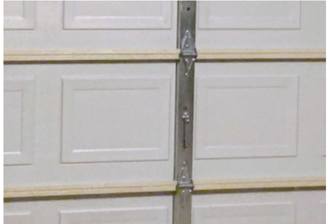
Figure B4: Sectional Door, Non-Insulated – Interior View Shows Hollow Panels
