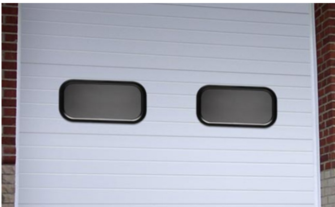
Figure B16: Sectional Door – Windows
