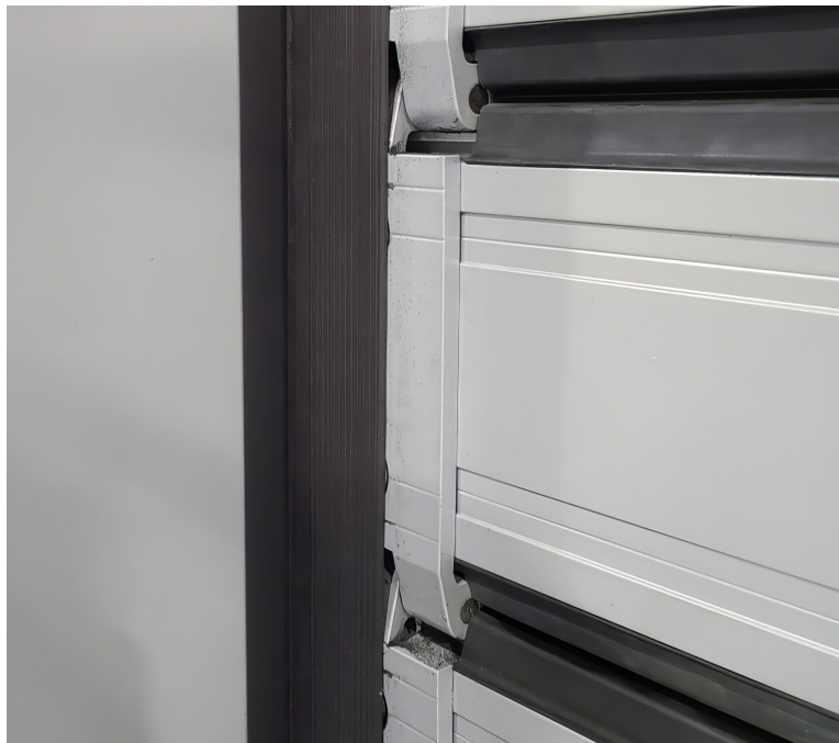
Figure B12: High Performance Door Interior Guide Seals – Good Condition
