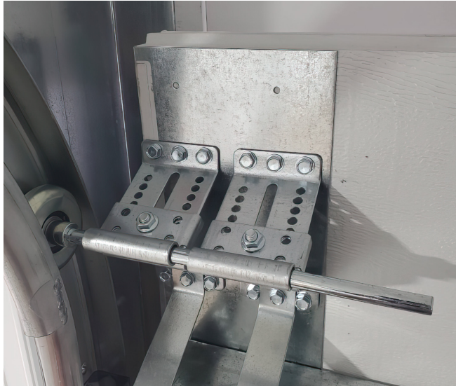
Figure B15: Sectional Door – Top Fixture
