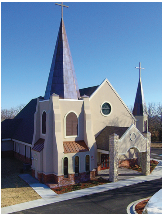
The Church of St. Francis Xavier in Sallisaw, OK is a metal building system with a 12:12 roof pitch, and additional built out structures in cold-formed steel.
