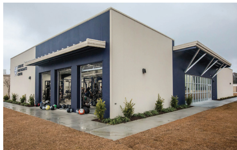
Charleston Southern University's new 8,000 sq. ft. athletic facility combines a 5,000 sq. ft. strength and conditioning center and a 3,000 sq. ft. meeting and office space, essential for recruiting as well as enhancing student-athlete wellness and the competitive experience.
