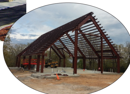
The Church of St. Francis Xavier in Sallisaw, OK is a metal building system with a 12:12 roof pitch, and additional built out structures in cold-formed steel.
