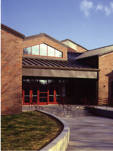
▲ Located in Lincoln, Ill., the classic brick facades of Lincoln Elementary School wrap the 33,500 sq. ft. structure built by P.J. Hoerr, Inc., and conceal a metal building system designed for the educational architecture.
